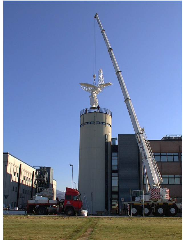
Fig. 1. The Polar 55C antenna to be installed over the top of the building of ISAC, in the Tor Vergata Area of the National Council of the Research.
